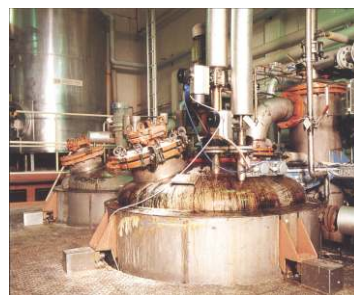
Batching Processes Reactors and Process Vessels
